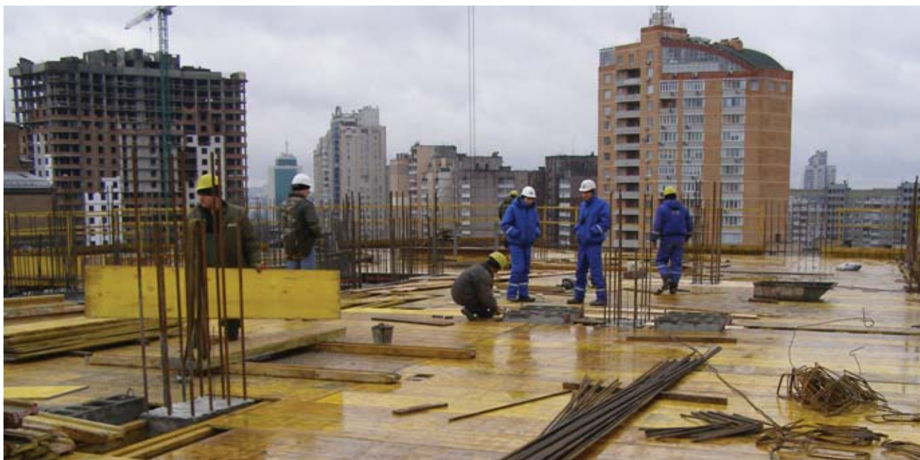
Installation of 3S wooden plate on slab formwork.
